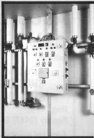
Control panels with mixing groups.
